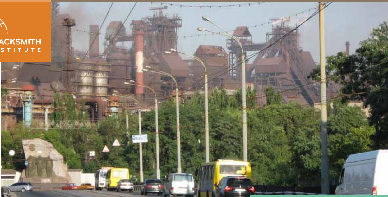
An Industrial steel processing complex
