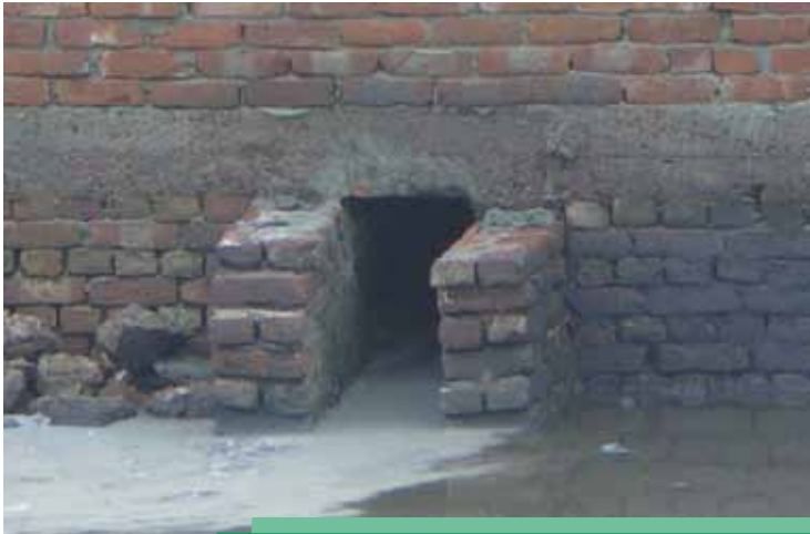
Tannery effluent flowing into surface waters
