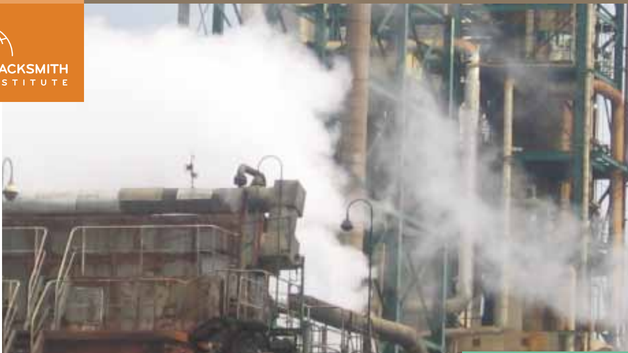
Chemical production facility
