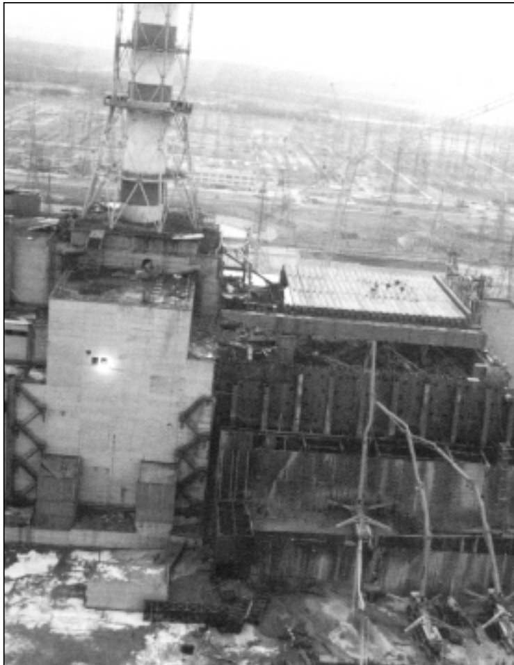
Construction of the reactor No. 4 sarcophagus
